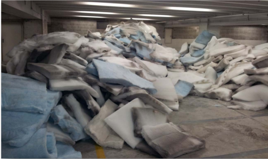
Removal of acoustic and thermal insulation
