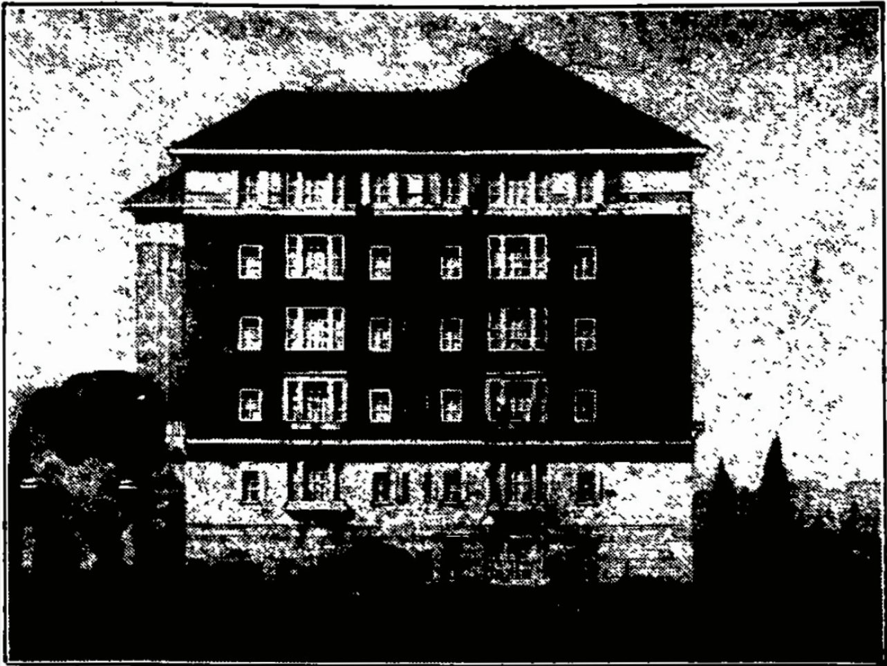
RESIDENTIAL FLATS IN PARNELL.— One of a group of four buildings to be erected on top of Parnell Rise, which are to be known as Mayfair Flats. The demolition of the old wooden houses on the site is now proceeding.
